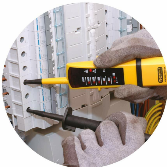
For socket wiring checks
